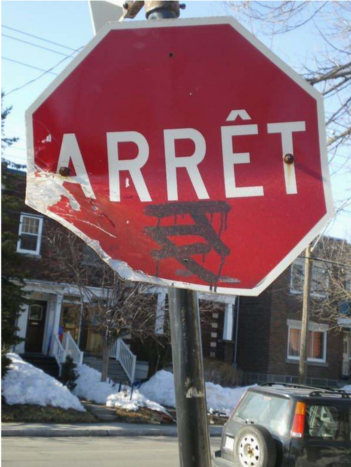
Figure 7: Sign 23-15-7. One of the most highly damaged signs.
