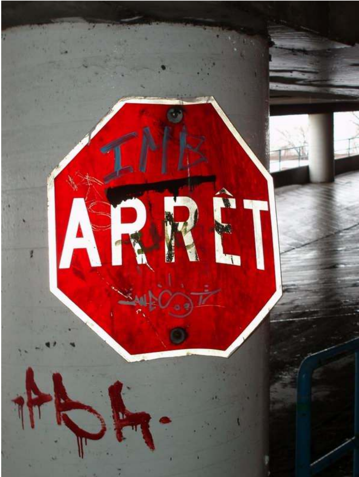
Figure 5: Sign 9-6-e. Example of high vandalism (intentional) and low wear (likely from car exhaust).
