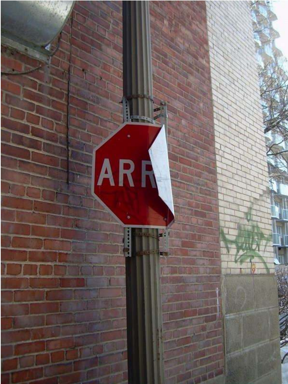
Figure 6: Sign 2-23-8. One of most highly damaged signs.
